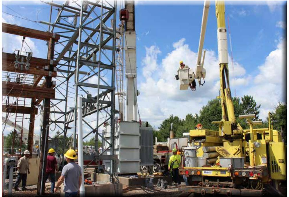
*Barron Electric crews worked together with Dairyland Power, PV Farmer and Utilities Plus to upgrade a transformer at the Johnson Timber Substation to help improve reliability.*
