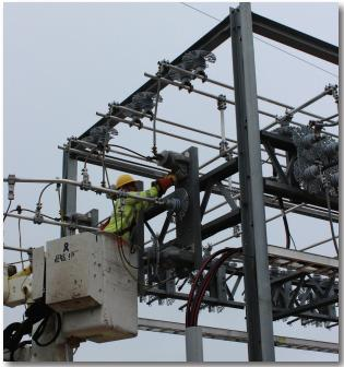
Pictured above: Lineman Aaron Holten puts some final touches on the North Wal Substation prior to energizing.
