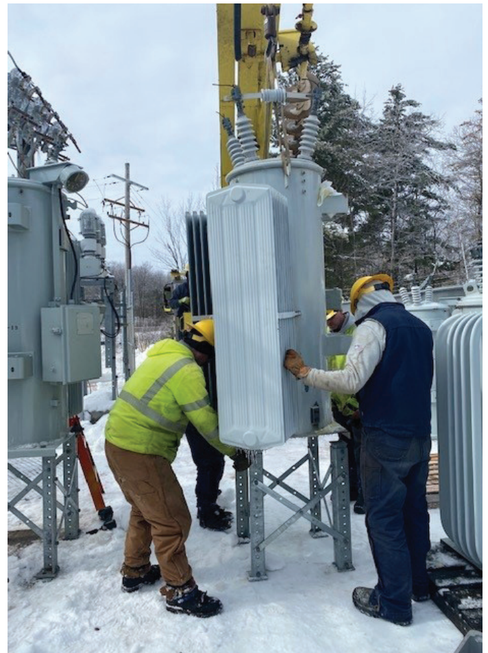
Line crews changed out a regulator at the Shell Lake Substation. Maintenance projects help to increase reliability and reduce outages, therefore, helping to reduce costs.
