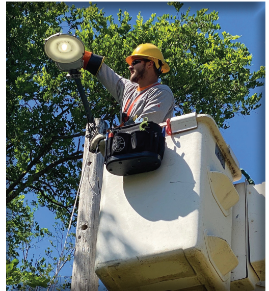
Lineman Trystin Adams installed an LED fixture into a dusk-to-dawn light.
