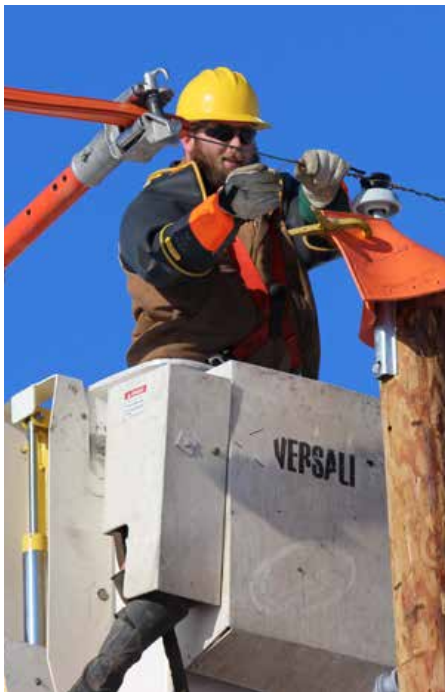
Lineman Mike Kroeze works on this upgrade.
