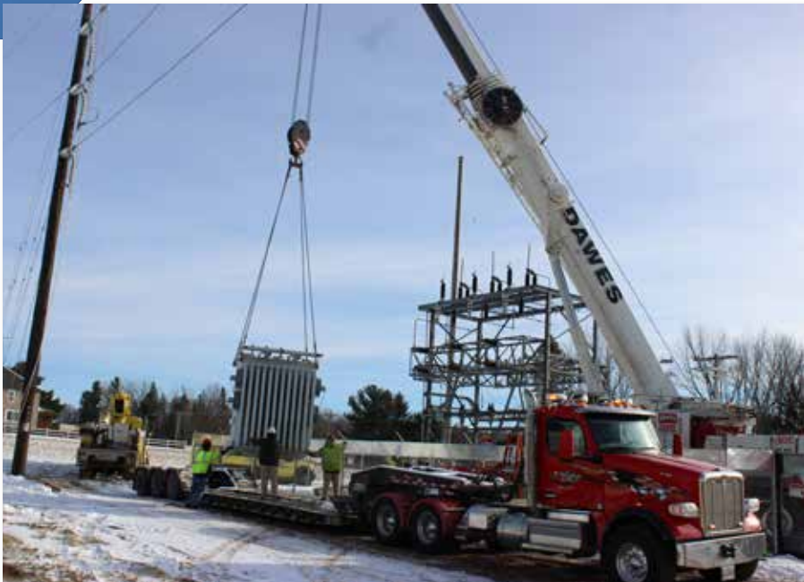
Crews upgraded the transformer at the Haugen Substation to help increase reliability.
